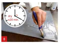
The surface must reach a thickness of 1 to 2 mm. Curing time of A1 is  $\pm$  20 minutes.
