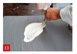
Apply a thin layer of A1 with a brush on the surface.
