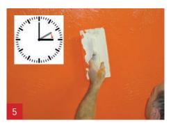
Use a stucco to create some structure (or any other tool) in the 1<sup>st</sup> A1 Plaster layer. Processing time is max. 1 hour.
