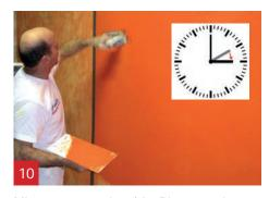
Mix a new quantity of A1 Plaster and apply a 2<sup>nd</sup> layer onto the surface and level it. You can use the same or a different colour.
