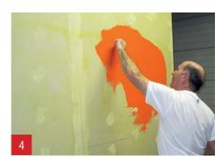
Apply a 1<sup>st</sup> layer of A1 Plaster using a stucco and level it (approx. 1 mm thickness).
